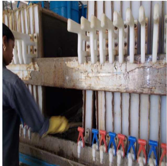
Fig. 7 - Filter press for dewatering of sludge slurry
