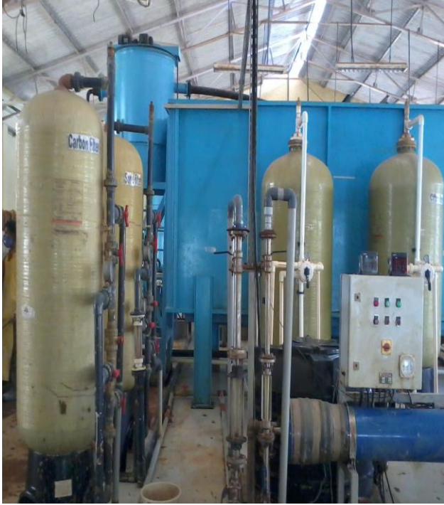
Fig. 8 - Dual media filter
