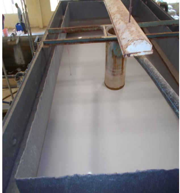
Fig. 5 - Clarifier without over flow through weirs
