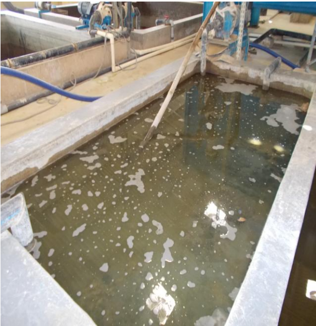
Fig. 6 - Sludge slurry storage tank
