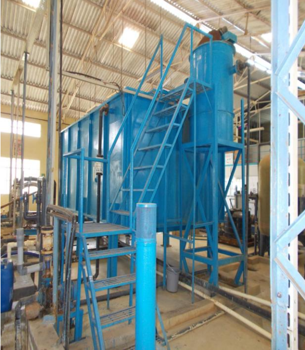
Fig. 5 - Clarifier without over flow through weirs
