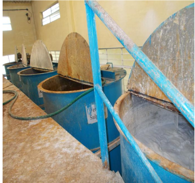
Fig. 2- Chemical dosage tanks
