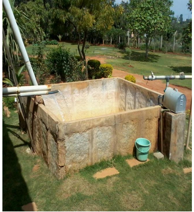
Fig. 9 - Treated effluent collection tank
